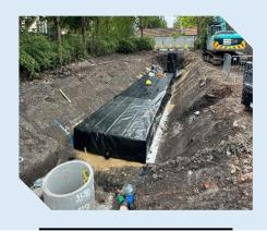
DXI undertook enabling works for a new Passivhaus student accommodation at Peru Street, Salford for Eric Wright Construction. The works comprised forming new entrances into site over dense existing services, removal and crushing to 6F2 of relic structures, chemical testing of suitability for retaining soils, engineering of piling platform for CFA and installation of drainage, all under an archaeological and UXO watching brief.
